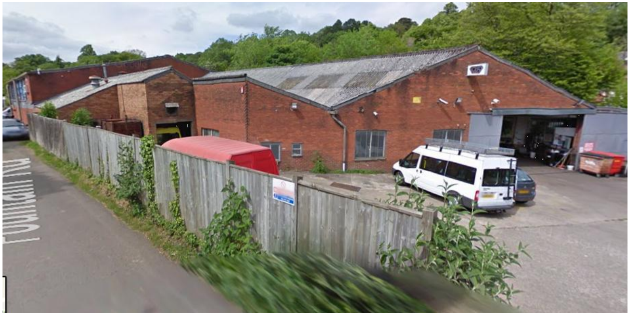
Figure 3 – View of rear of building from Fountain Road
